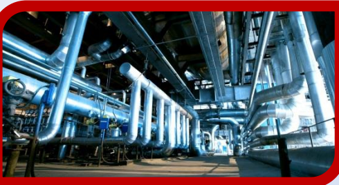
Constructing & equipping facilities for Seaport and terminal
