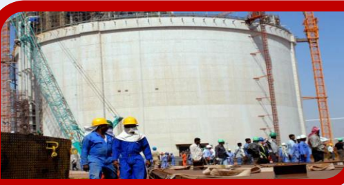
Equipping of oil and gas tanks
