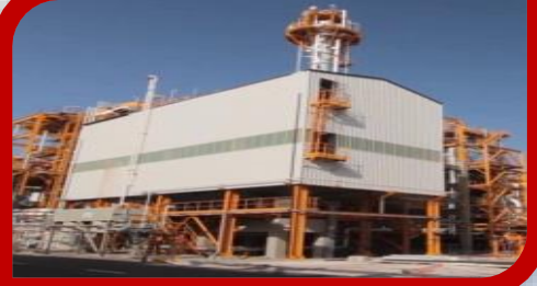
Implementation of facilities & Steel buildings
