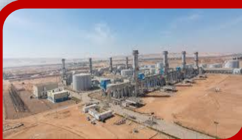
Construction & processed oil facilities & refineries
