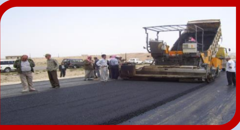
Incision and paving of roads
